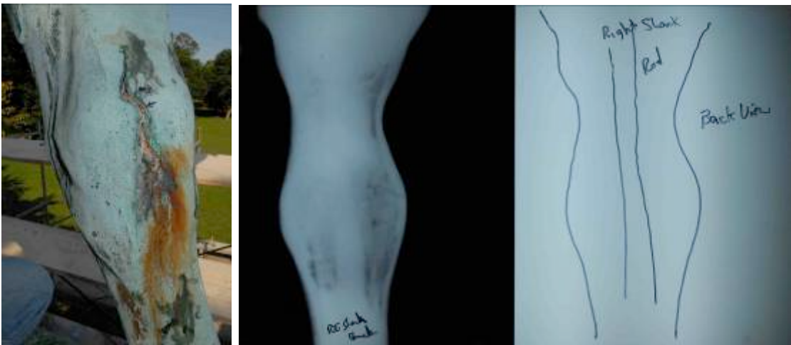
Fig. 10. Detail of the proper left front leg of the horse. The image on the left illustrates external structural problems caused by deterioration of the internal ferrous armature and concrete fill. The white seen inside the leg was proved to be concrete (MVA analysis – see attached report). The material deposited under the crack is rusty in color and comes from decomposing ferrous reinforcement clearly visible in the x-ray image in the middle and drawing on the right. This long crack was created by freeze and thaw cycles, expansion of deteriorated concrete material and expansion of ferrous corrosion products. Iron corrosion products and core material leach out.
