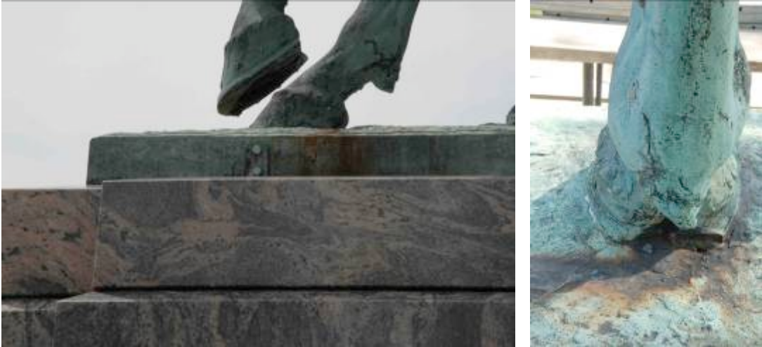
Fig. 2. Detail of the proper left side of the base - showing the bracket, and iron stain leaching out from the inside of the horses leg.
