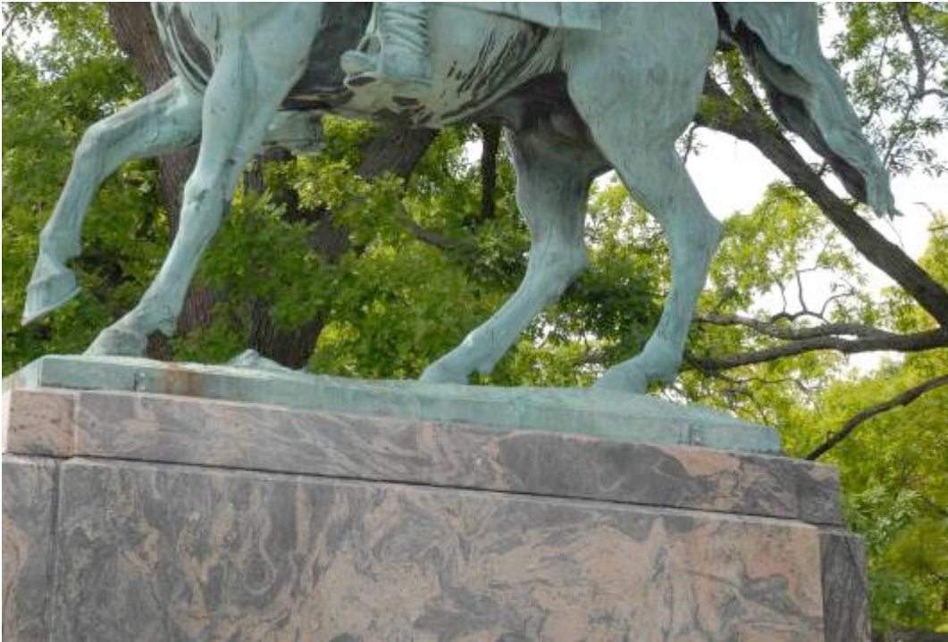
Fig. 1. Proper left side view. The entire surface is corroded - disfiguring green, and black streaking. Please notice the two brackets attaching the base of the bronze to the stone. Please also notice the rusty stain at the front of the bronze base.
